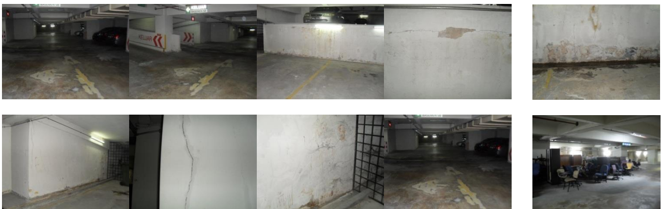
Figure 3.3: Photo of General Condition at Basement 5 - 6
