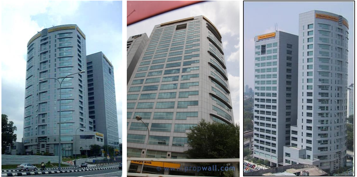
Figure 3.1 General views at DataranMaybank, Bangsar
