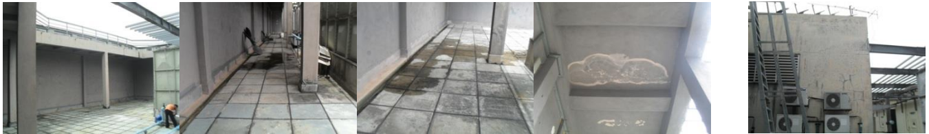
Figure 3.12: Photo of General Condition at Rooftop Tower C level 23
