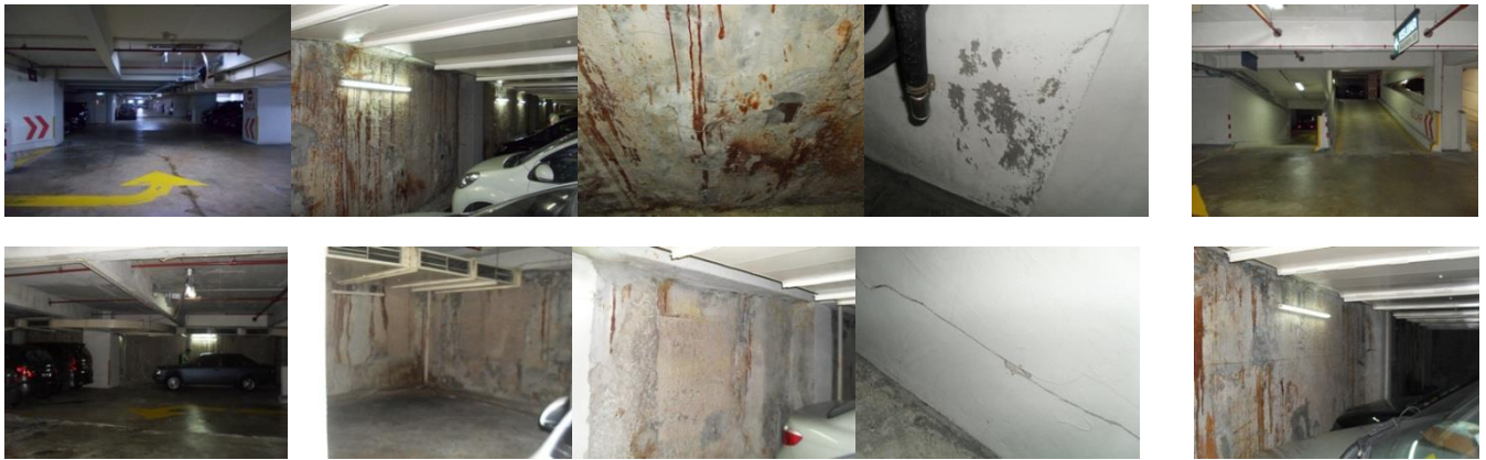
Figure 3.1: Photo of General Condition at Basement 1 - 2
