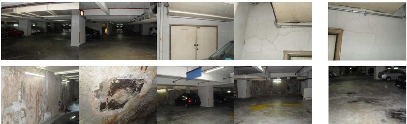
Figure 3.2: Photo of General Condition at Basement 3 - 4
