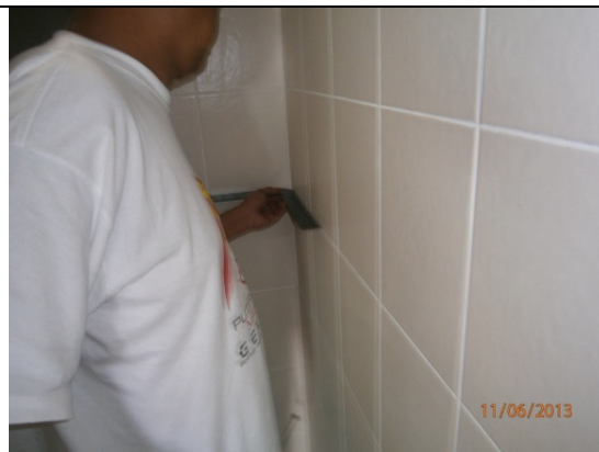
Figure 3.12 : Assessment Using L-Square
