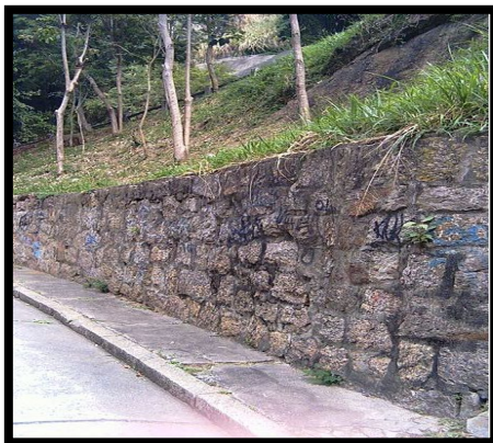
Figure 2.7 show the face of retaining wall
