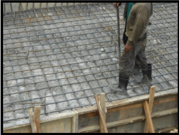
Figure 3.18 show the installation of steel bar
