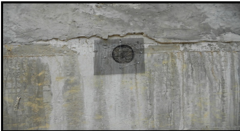
Figure 3.33 show the installation of crusher run on weep hole
