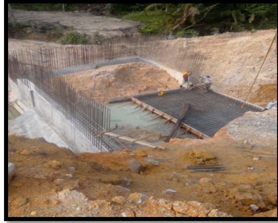
Figure 3.24 show formwork on base retaining wall
