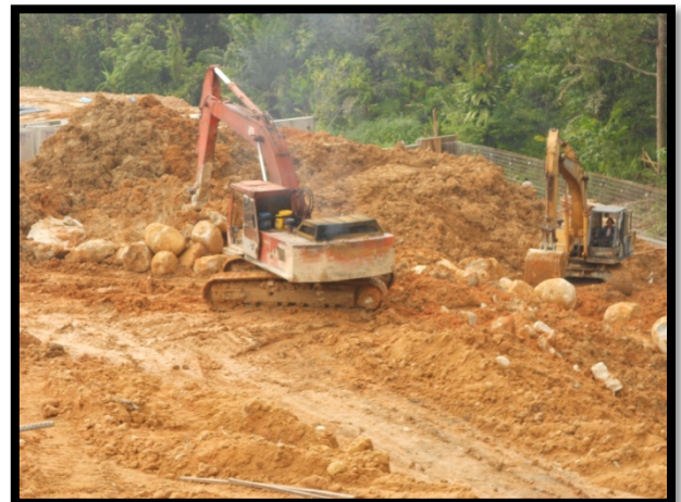
Figure 4.4 show the rock was found too many
