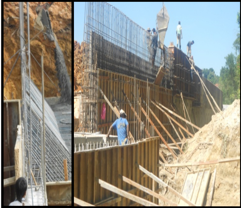
Figure 3.26 show c Figure 3.27 show the concrete test report
