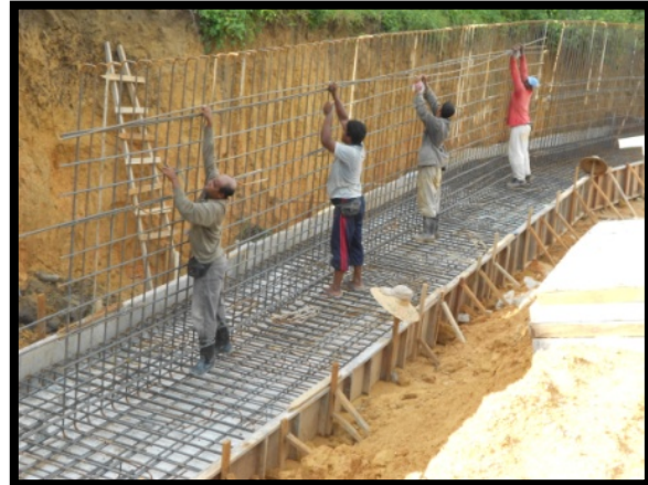
Figure 3.19 show the spacing of steel bar
