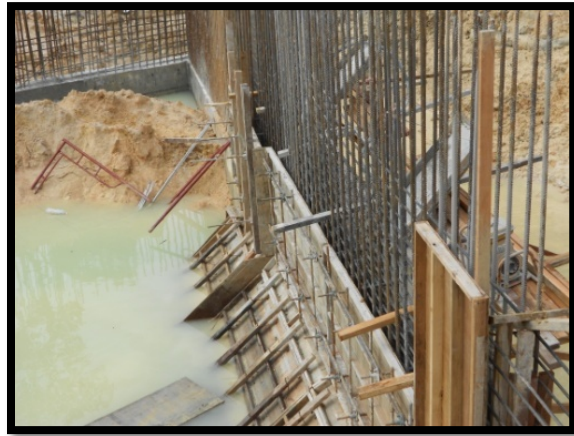
Figure 3.22 show the installation of weep hole
