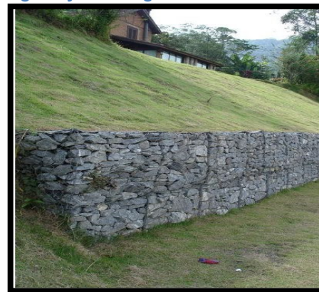
Figure 2.8 show the type of gravity retaining wall
