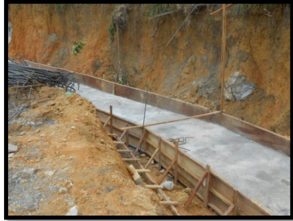
Figure 3.17 show the lean concrete on base retaining wall
