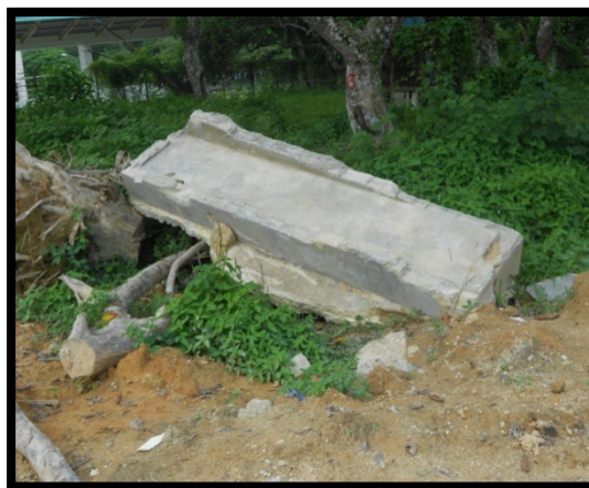
Figure 3.6 show the beam that have been demolish
