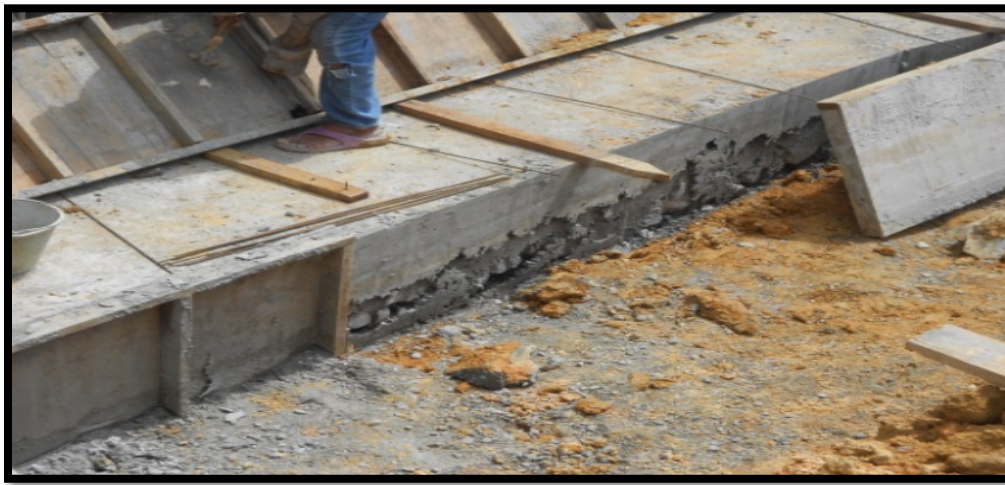
Figure 3.30 show the removing formwork
