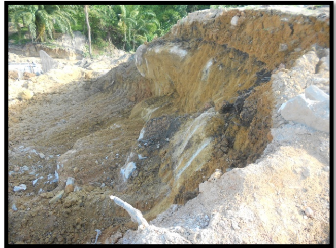
Figure 3.15 show the rock have been found
