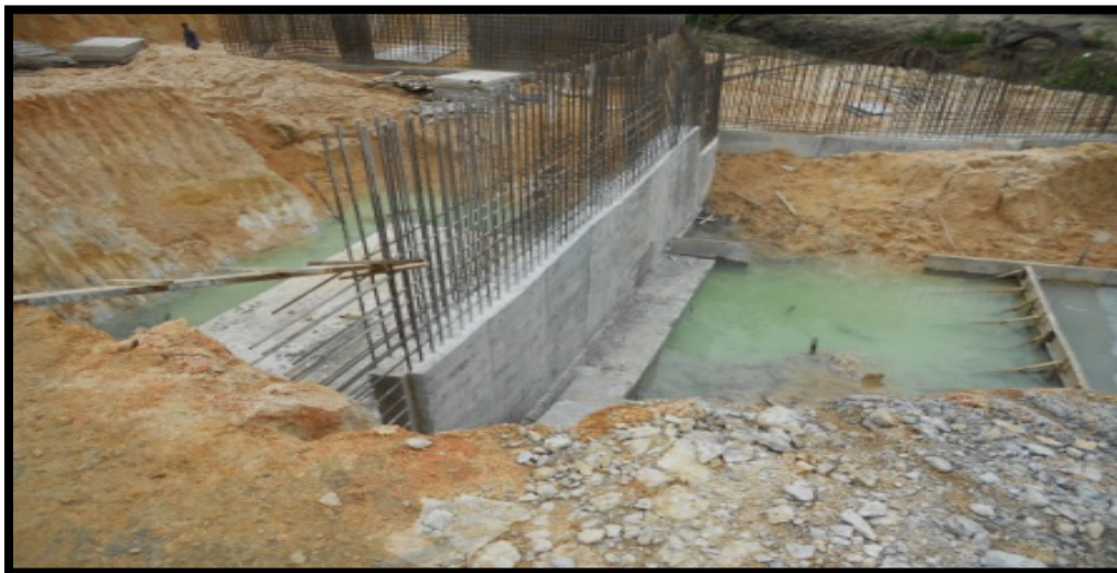
Figure 3.31 show the retaining wall that have been complete remove with formwork
