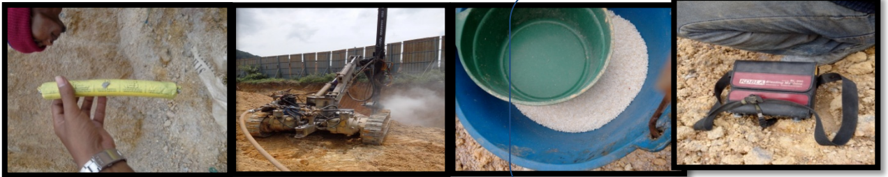
Material use: dynamite, drilling machine, seed, blasting machine, electric detonator.
