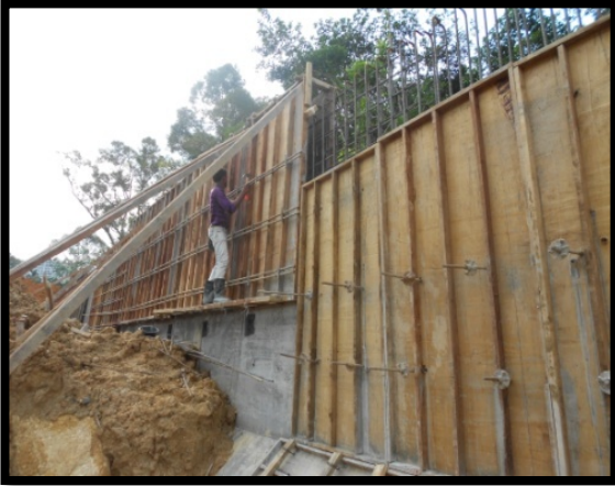
Figure 3.23 show the installation of formwork
