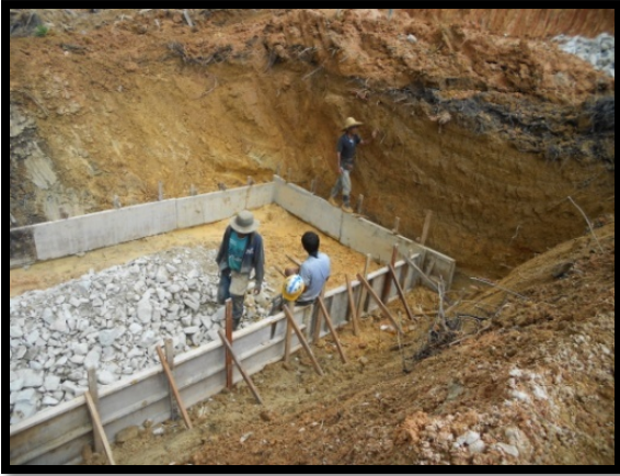
Figure 3.16 show filling of hardcore
