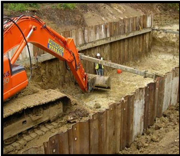
Figure 2.1 show the excavation of base retaining wall
