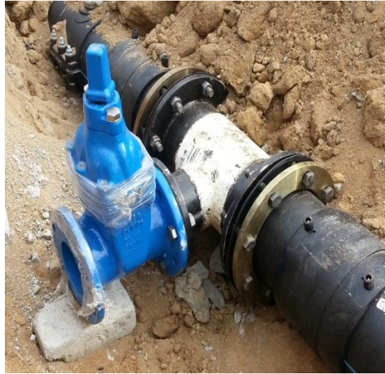
Figure 4.15: Installation T-Valve/Gate Valve
