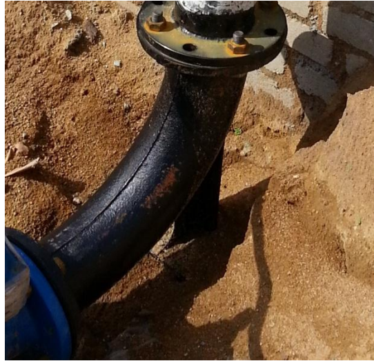
Figure 4.8: 45° bend fitting
