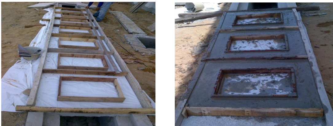
Figure 4.10.2 Drainage Cover Work
