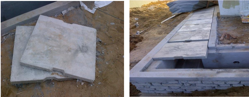
Figure 4.10.3 Drainage Cover
