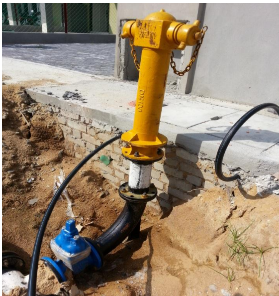
Figure 4.16: Installation of Hydrant
