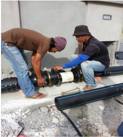
Figure 4.14: Installation Tee
