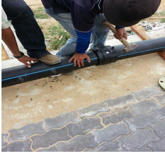
Figure 4.11: Installation electro fusion coupler
