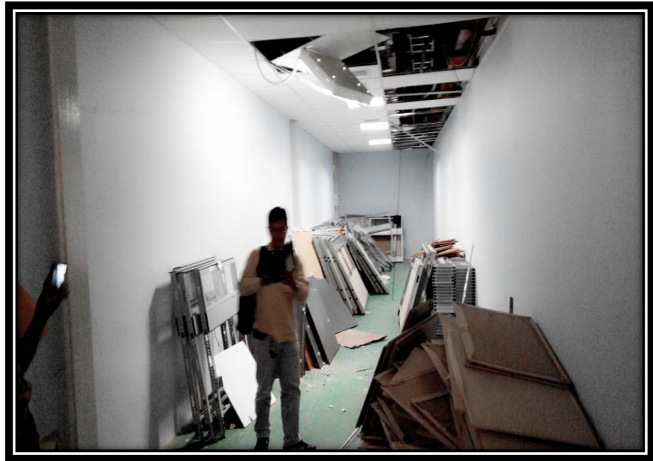
3.5 The picture about the ceiling that should replaced
