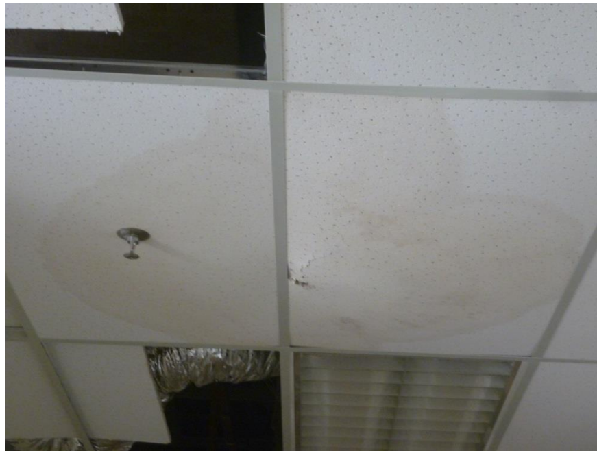
Figure 3.3 Shows the broken ceiling
