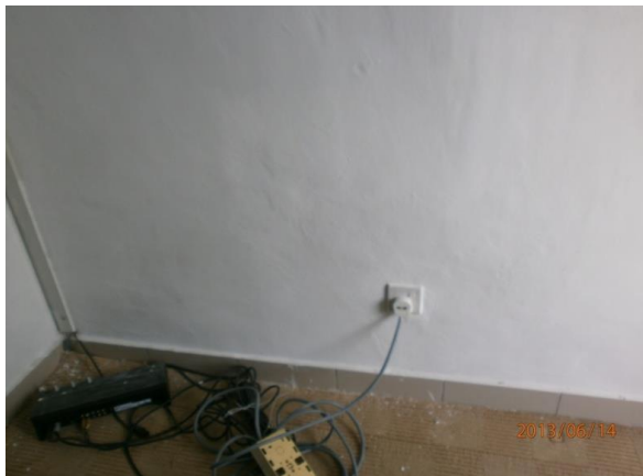
Figure 3.7 show the crack inside the building has been repair
