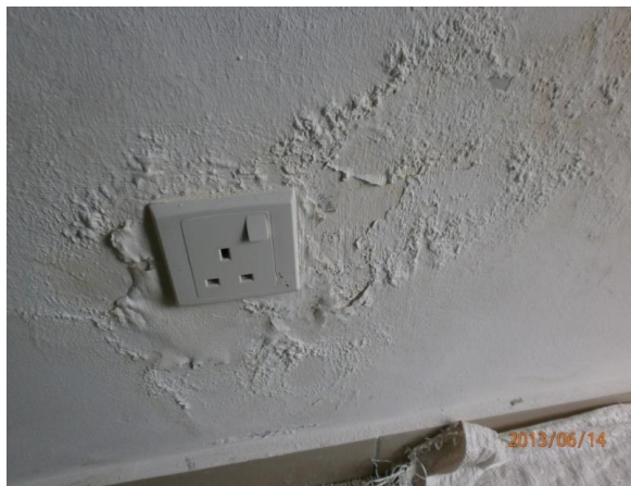
Figure 3.4 Show the peel of paint ( dampness ) inside the building
