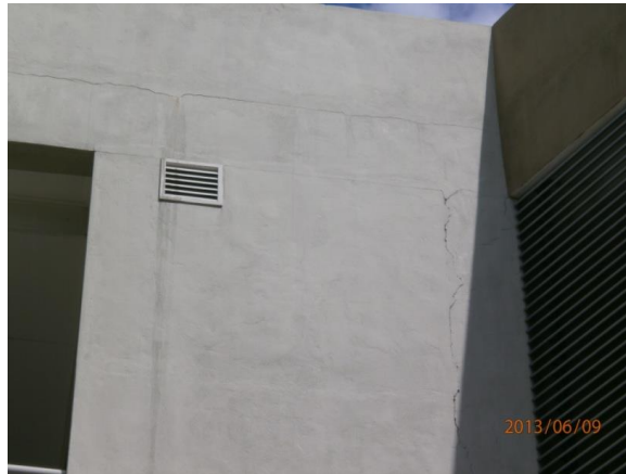
Figure 3.3 Show the crack outside the building
