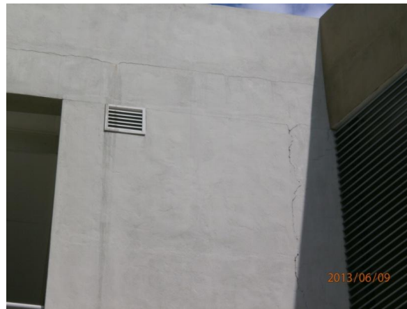
Figure 3.6 : Crack Outside
