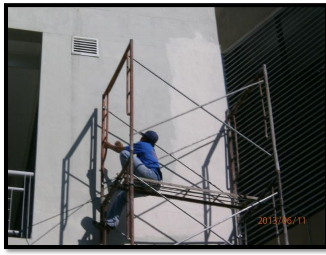
Figure 3.9 plastering work
