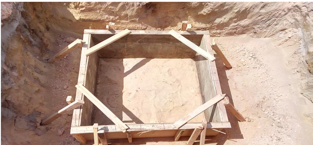
Photo 3.7.2: formwork for pad footing
