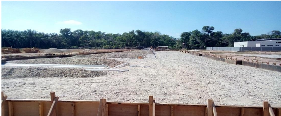
Photo 3.6.3.2: laying hard core (block B)
