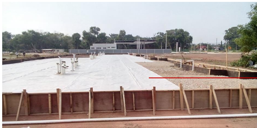
Photo 3.6.5.1.: installation plastic layer (block B)
