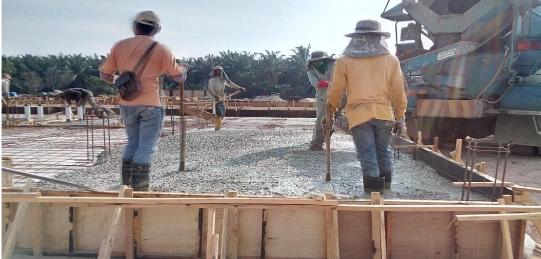
Photo 3.6.8.3: laying concrete
