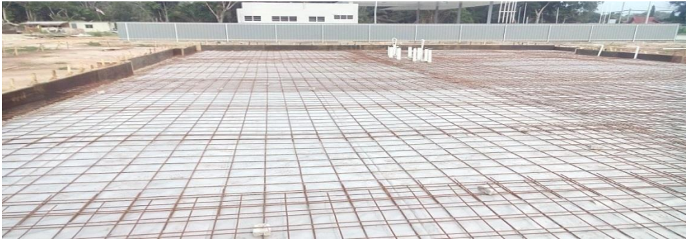
Photo 3.6.6.1: Installation BRC A7 at Block B (left elevation)
