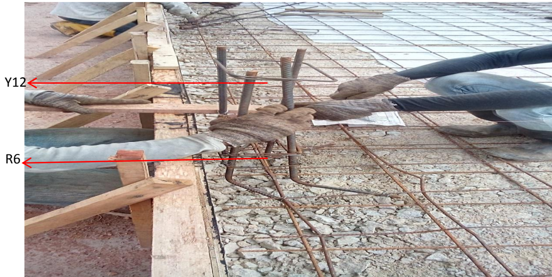
Photo 3.6.7.1: installation column stump steel
