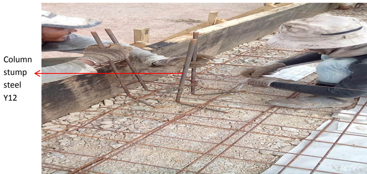
Photo 3.6.7.2: installation column stump steel
