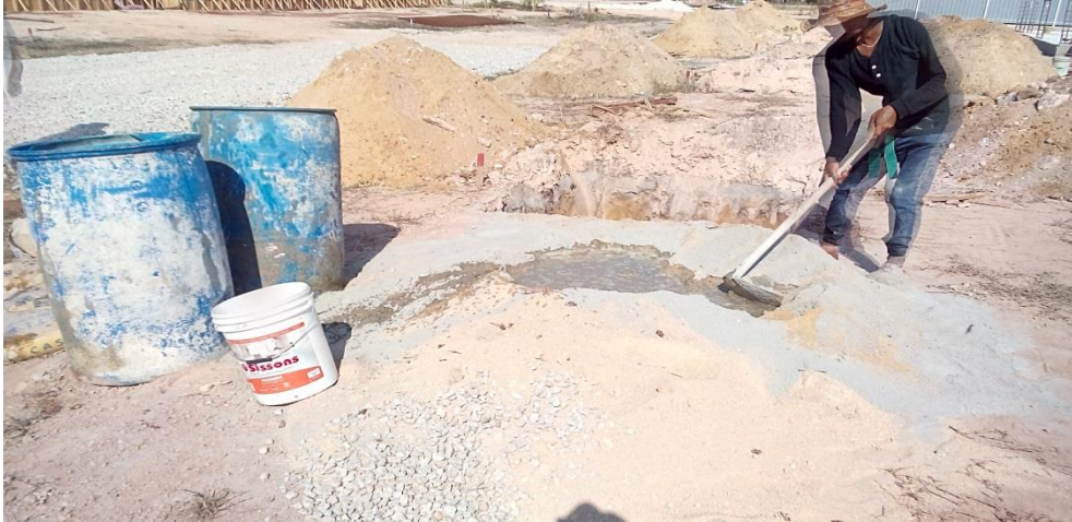
Photo 3.7.3: concrete in-situ for lean concrete
