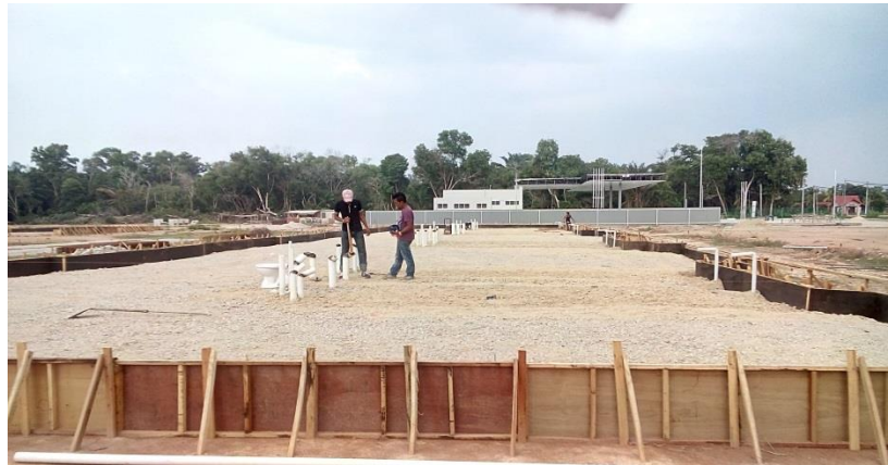
Photo 3.6.4.1.: spray anti-termite (block B)
