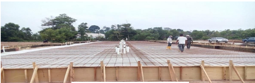
Photo 3.6.6.2: Installation BRC A7 at Block B (right elevation)
