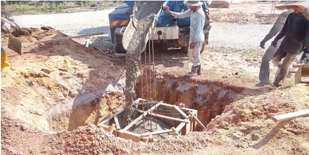
Photo 3.7.7: concrete work (pre-cast)
