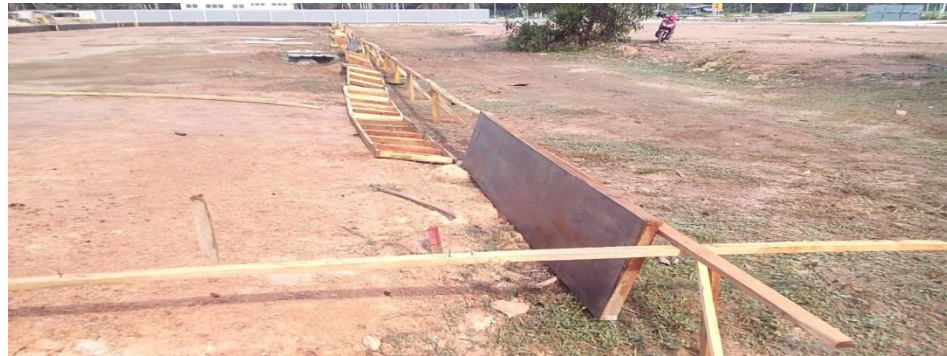
Photo 3.6.2.2: formwork ground beam (block B)
