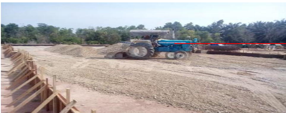
Photo 3.6.3.1: laying hard core (block B)
