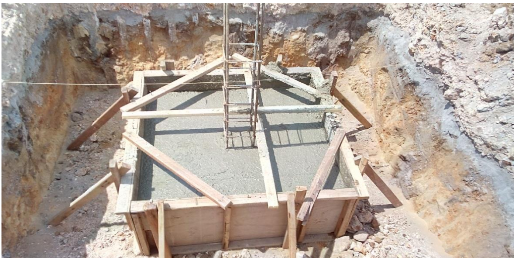
Photo 3.7.8: laying concrete
