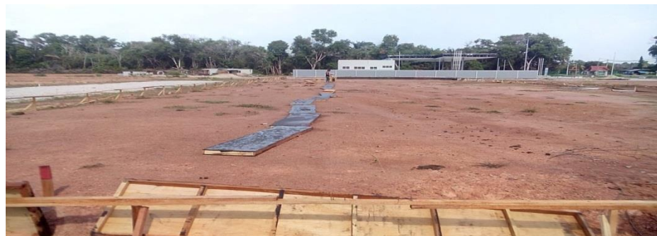
Photo 3.6.2.3: formwork ground beam (block B)
