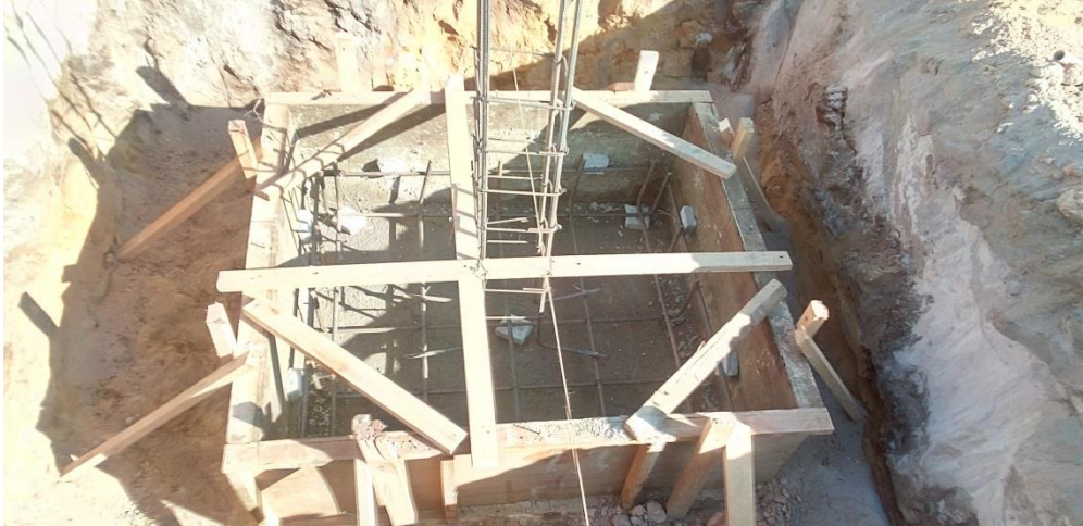
Photo 3.7.5: installation column stump steel
