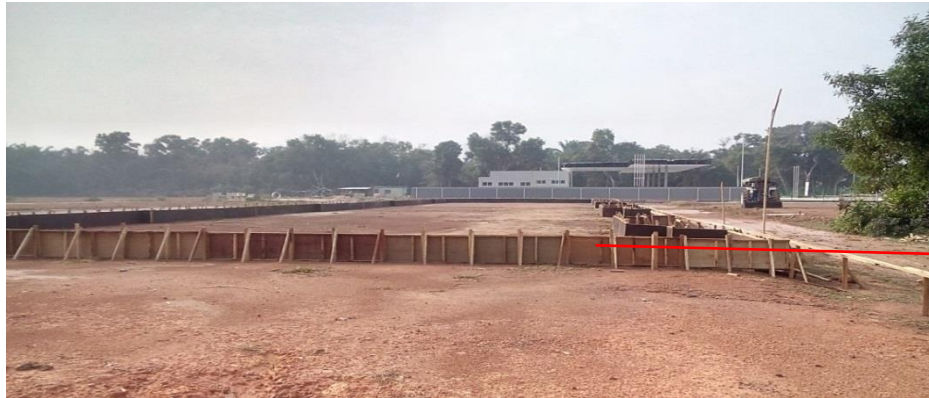
Photo 3.6.2.4: formwork ground beam (block B)
