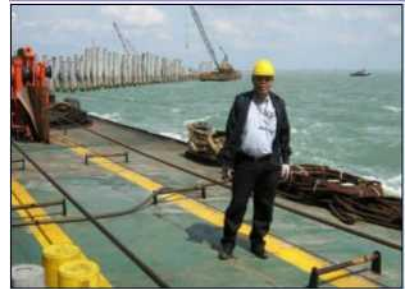
Assoc. Prof. Malit auditing a piling project in Port Dickson
