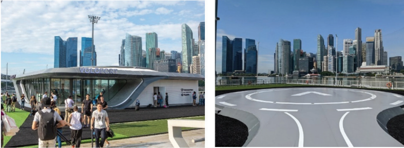
Figures 1. (left) & 2 (right): Exterior View Towards the Entrance of the Terminal, and the View of the Take-off and Landing Platform Equipped at the VoloPort
