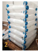
Figure 17: Process of Producing the Columns. (1) Doubled-Bottles Attached by Elastic Straps. (2) Plastic Straps as Stiffeners Source: Author
