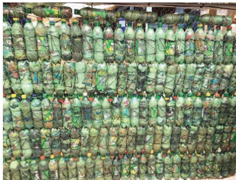
Figure 6: Bottle inCconstruction in Guatemala (Source: tammyblomsterberg.com)
