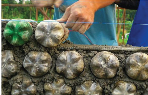
Figure 5: Bottle Bricks as Bricks in Construction (Source: thehomestead.guru)
