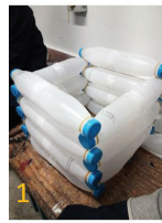
Figure 17: Process of Producing the Columns. (1) Doubled-Bottles Attached by Elastic Straps. (2) Plastic Straps as Stiffeners Source: Author
