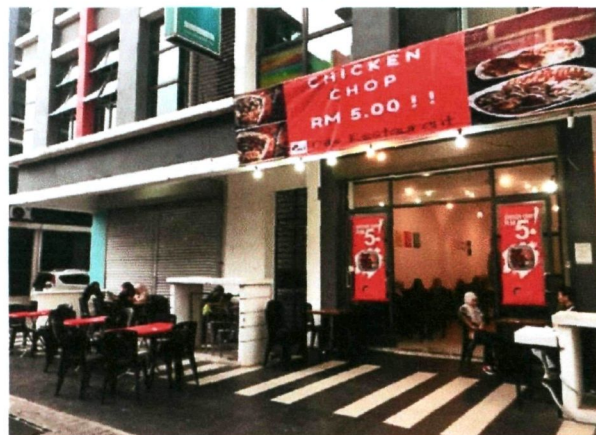
Figure 1: The main door for Dill's Restaurant
