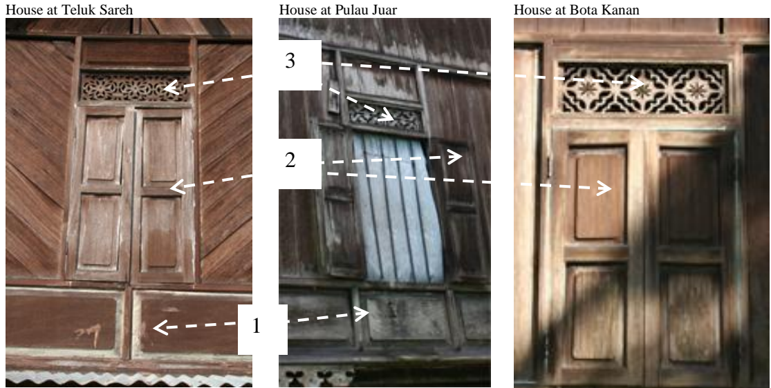
Legend: 1. Panel papan (dado wall), 2. 'Tingkap sekerat' (Half window), 3. 'Atas tingkap' (top of window). Photo 8: Wall and window component of houses built by Chinese tukang.
