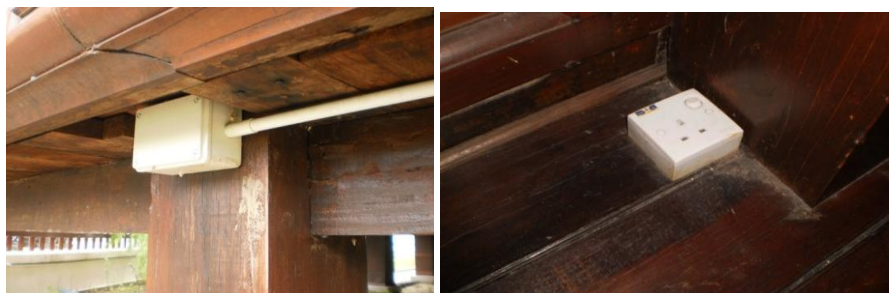
Photo 12 (a) The distribution board installed underneath the floor board. (Mulong Old Mosque) and (b) The power point is installed on the floor surface. (Mulong Old Mosque).
