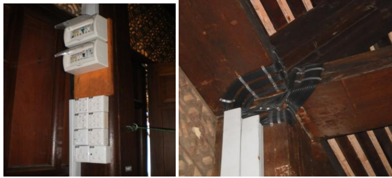
Photo 13 (a) The electrical fittings' switches is placed at one place. (Mulong Old Mosque) and (b) The electrical trenching conduits for electrical fittings are laid on the top of roof beam. (Mulong Old Mosque).
