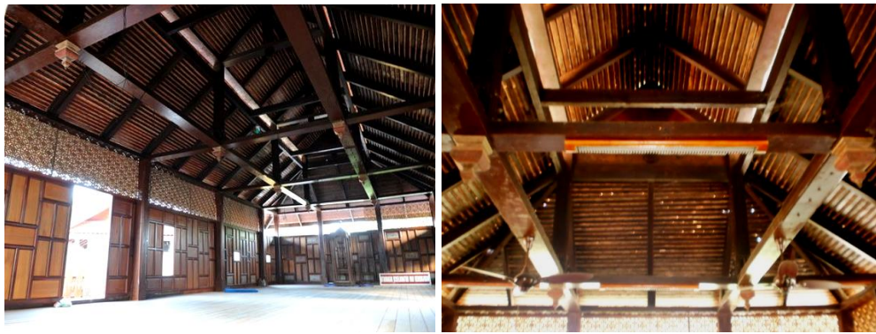
Photo 9 (a) and (b): Exposed roof structure. The roof structure is made of high quality Chengal wood. The exposed roof structure shows the beauty and uniqueness of Malay traditional building construction.
