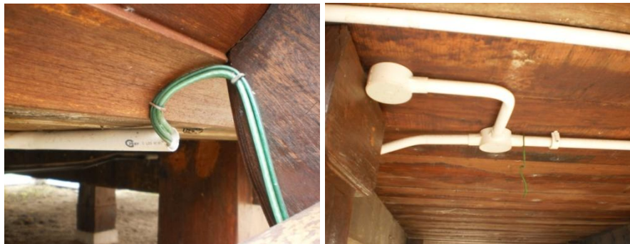
Photo 11 (a) and (b): The trenching of electrical conduits for power point is laid underneath the floor board to avoid visibility of the trenching conduit (Mulong Old Mosque).
