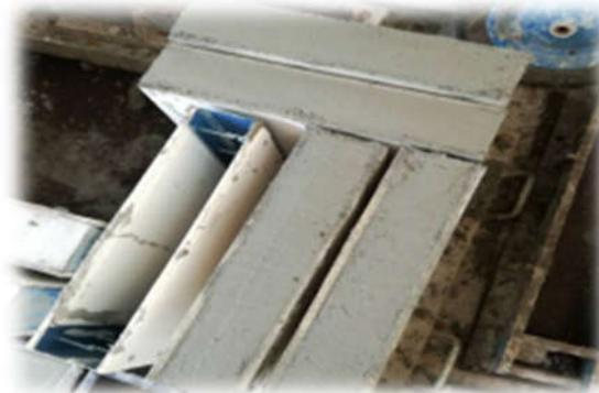
Figure 2: Filling the panel with foamcrete core
