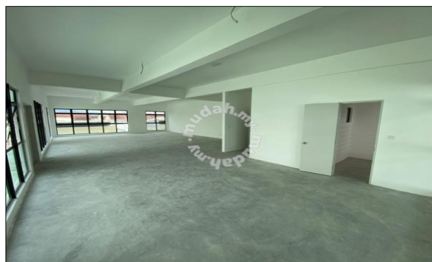
Figure 2: Inside the Building
