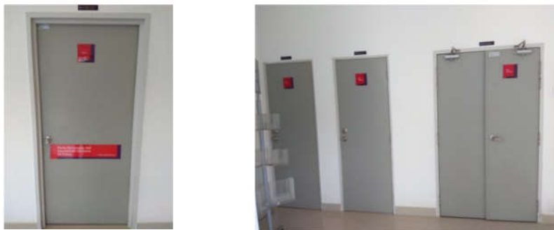
Figure 4: (a) Single Fire door (b) Double leaf door of fire door
