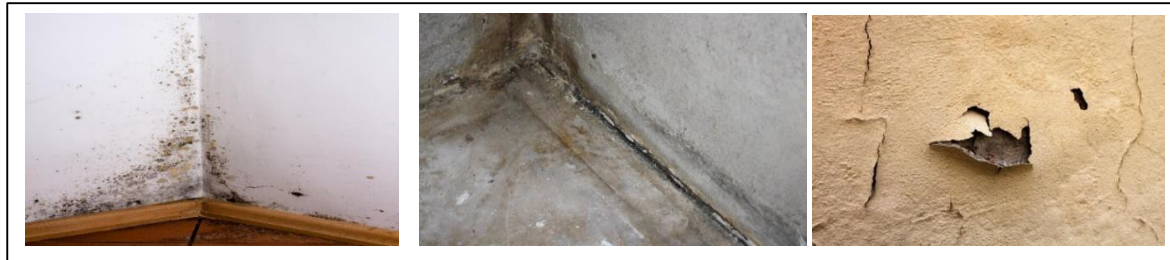
Figure 2 The building defects occur at building due to humidity
