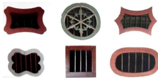
Figure 4 Simple Carved Timber Air Vents of Shophouses. Source: Author Tan, 2015
