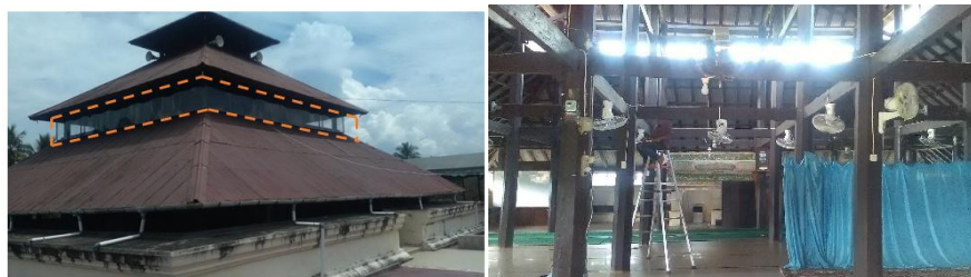
Figure 7 The roof aperture sealed with plastic and the fans installed and attached to the wooden beams
