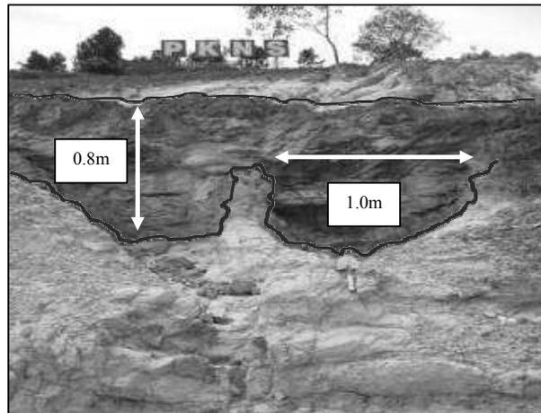
Plate 1: Raveling of the slope
