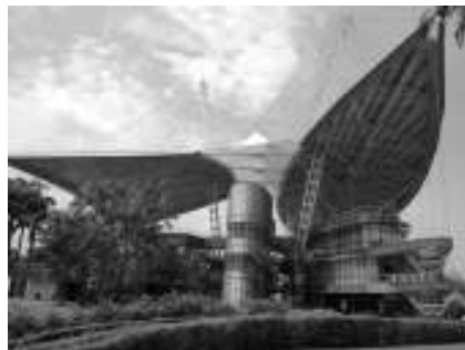
Figure 4: The Guthrie building can be considered as the pioneer modern building in the tropic region to fully consider on implementing sustainable design issues through the bioclimatic approach design philosophy. The building is fully glazed for maximum views out and natural lighting.(Source: Roslan Hj Talib (2011)
