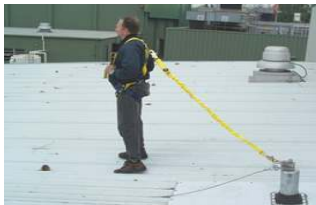
Photo 2: Flat roof with anchorage point for workers to suspend lanyard of their safety harness as fall from height protection Source: http://www.anchorsafe.com.au
