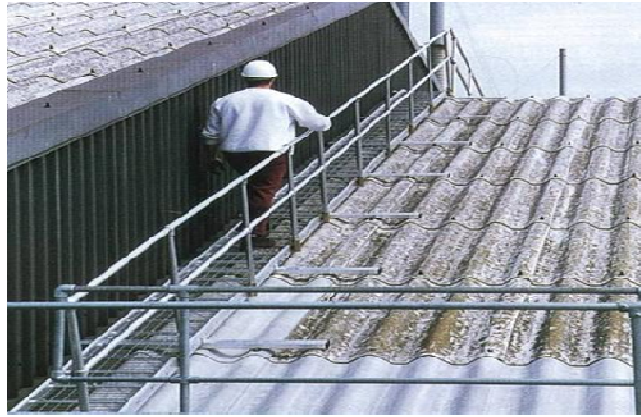
Photo 3: Walk able route with handrails at steep and brittle roof Source: https://millrace.uoregon.edu/uopress/index.cfm
