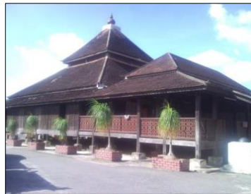
Figure 1: The Three-Tiered Pyramidal Roof Form of Kampung Laut Mosque
