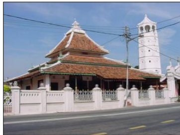
Figure 9: The Three-Tiered Pyramidal Roof Form of Tengkeria Mosque
