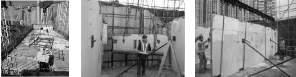
Figure 6 Trial Run of Demolition
