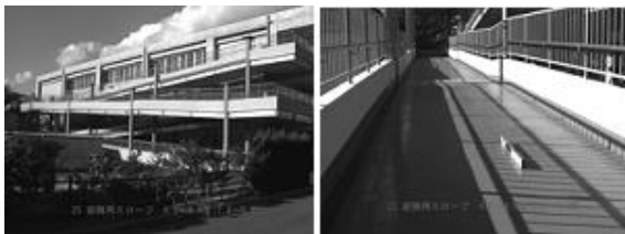
Figure 5 Overview of slope surface route
