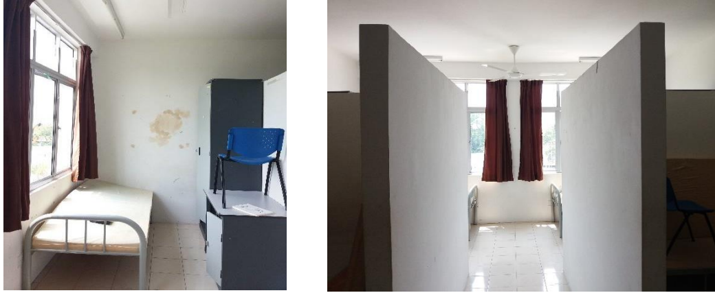
Figure 3 Existing condition of the case study room
