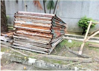
(a) Scaffolds are not properly stored
