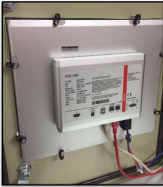
Figure 5: PC-based controller CP2612 (Back view).
