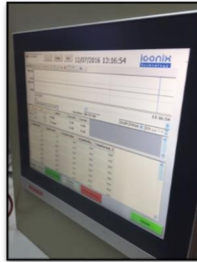
Figure 6: HMI SCADA display.
