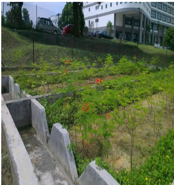
Figure 4. Bioretention System in UNITEN, Putrajaya Campus
