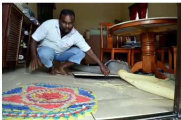
Figure 3: Twelve houses in Kampung Tersusun Buntong, Ipoh were damaged when the foundation of their houses started sinking. Image copyright Bernama (2014)
