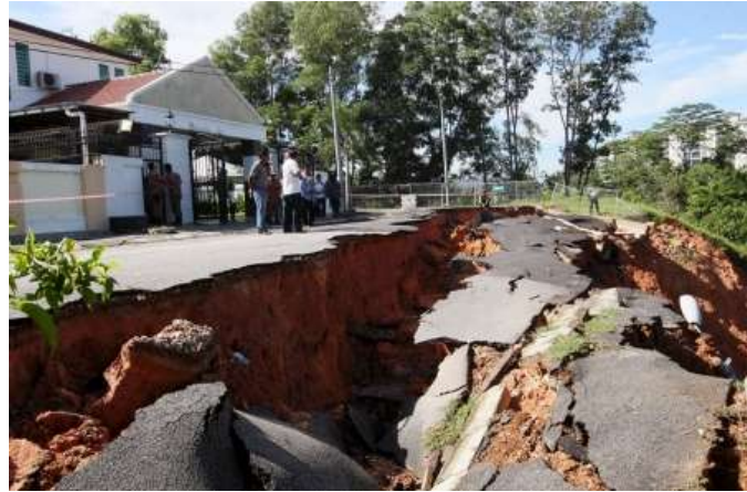
Figure 4: A Landslide hits Gerbang Meru Indah in Ipoh. Image Copyright, Manimaran(2014).
