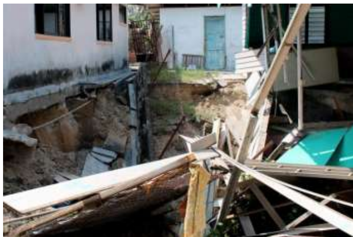
Figure 2: A sinkholes caused a five-meter deep crack developing inside a wooden house in Ipoh. Image copyright, The Star Online (2014).
