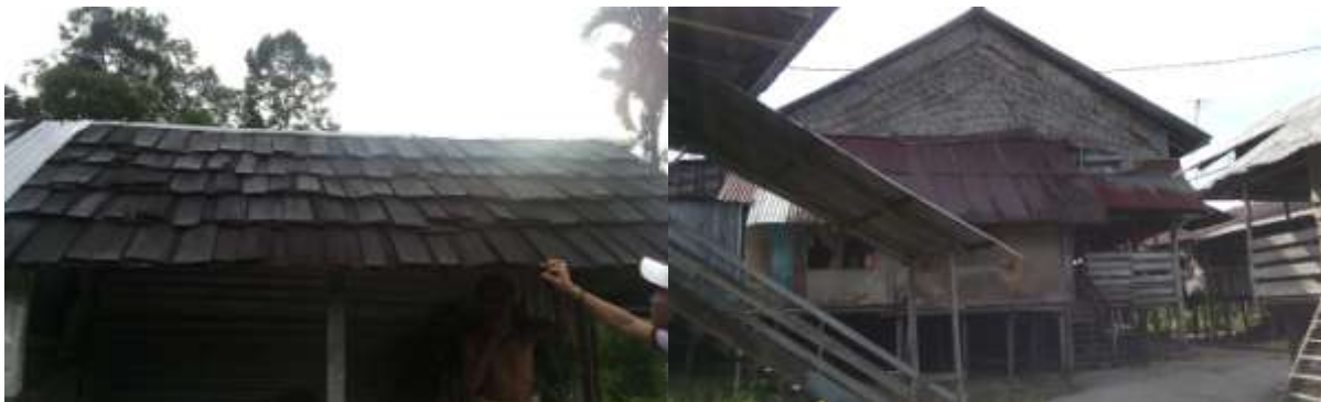
Figure 4: Timber shingles and sago/palm thatched for roofing. Image Copyright, Victoria (2015).
