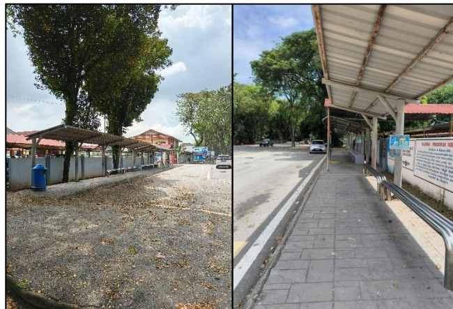
Plate 5.52 Drop-off Zone Adjacent to Bus Stop at SK Seksyen 24
