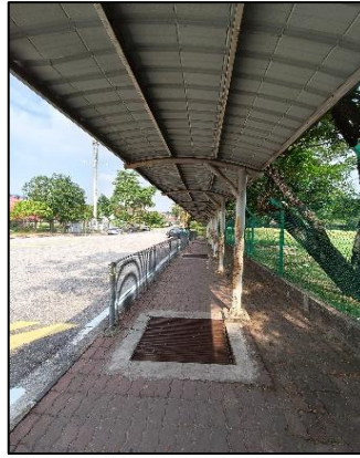
Plate 5.71 Pedestrian Walkway at SK Jalan U3
