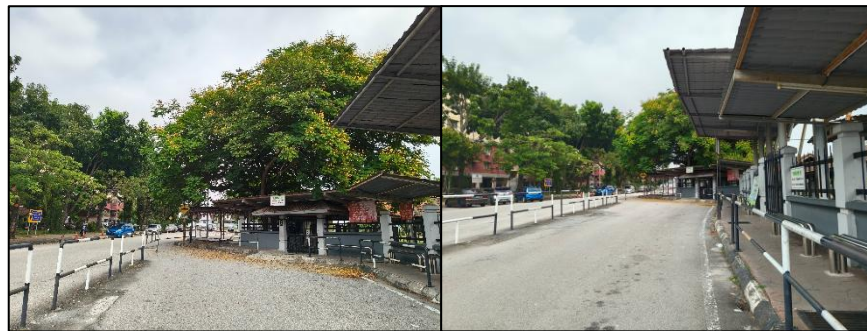
Plate 5.9 Drop-off Zone Adjacent to Bus Stop at SK Seksyen 7
