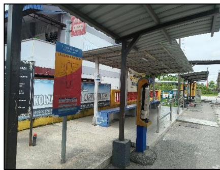
Plate 5.65 Narrow Bus Stop Lacking Lay-by Area at SK Padang Jawa
