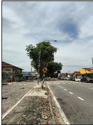
Plate 5.54 General Street Lighting at SK Seksyen 24
