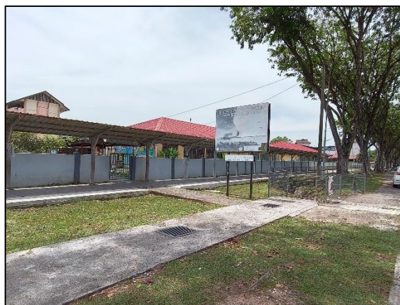
Plate 5.56 Sheltered Walkway at SK Seksyen 24
