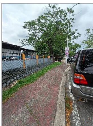
Plate 5.30 Lack of Fencing at SK Seksyen 17
