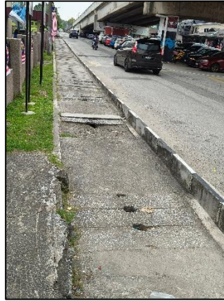
Plate 5.59 Narrow Walkways at SK Padang Jawa
