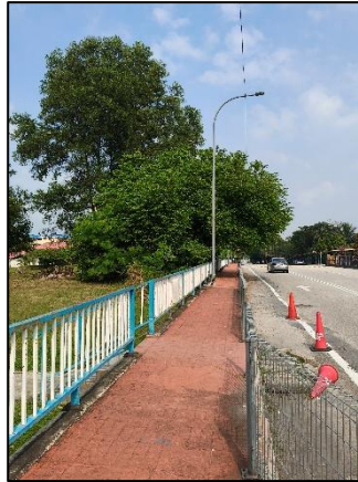
Plate 5.78 Street Lighting at SK Jalan U3
