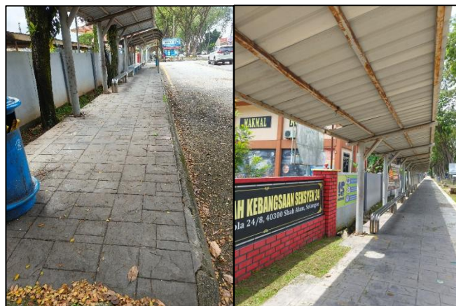
Plate 5.46 Wide and Continuous Pedestrian Walkway at SK Seksyen 24
