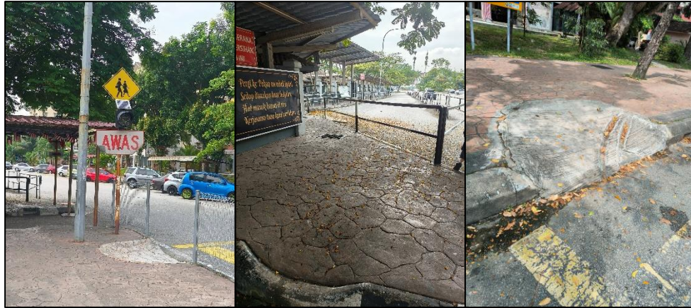
Plate 5.4 Curb Ramp Enhancing Accessibility at SK Seksyen 7
