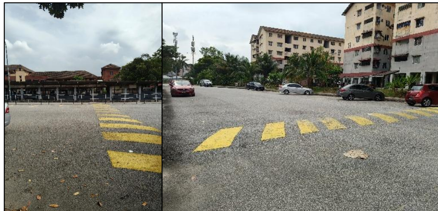
Plate 5.7 Speed Hump for Vehicle Speed Reduction at SK Seksyen 7
