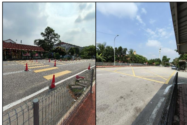
Plate 5.74 Clear Crosswalk Near Entrance at SK Jalan U3
