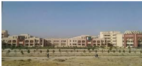
Figure 4. Engineering Faculty Building
