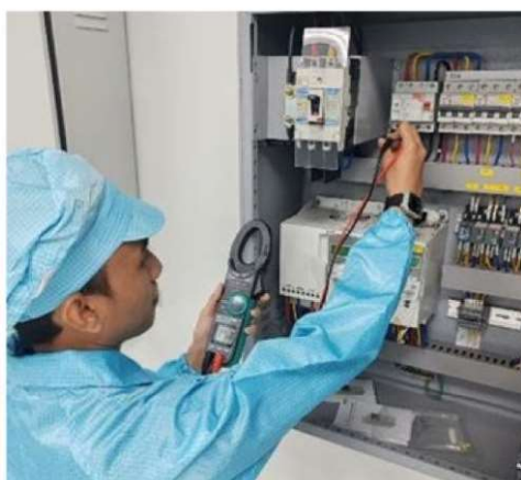
Figure 3: Taking RCCB Voltage Reading During Machine Troubleshooting
