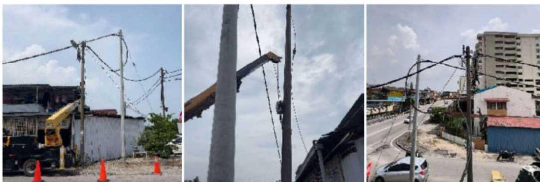
Figure 2: Cable Routing Process
