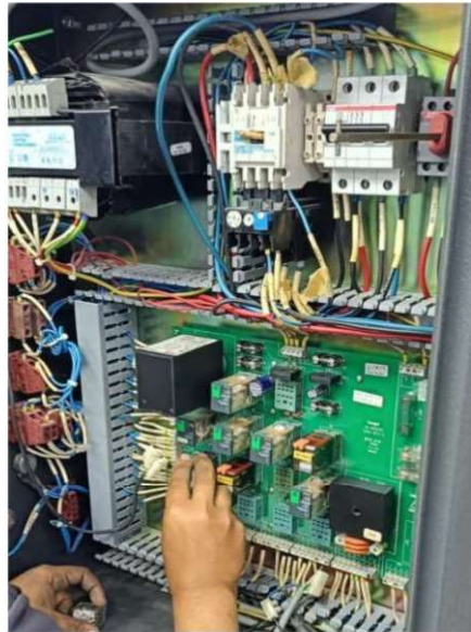
Figure 2: Replace Faulty Relays of the Clinching Machine
