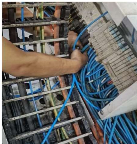
Figure 4: Diagnosing Air Leakage in Pneumatic Systems
