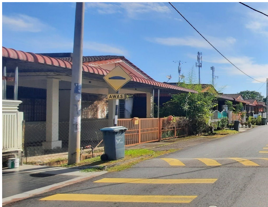
Figure 4.1: Only a few front areas of the housing units remain as provided by the developer
