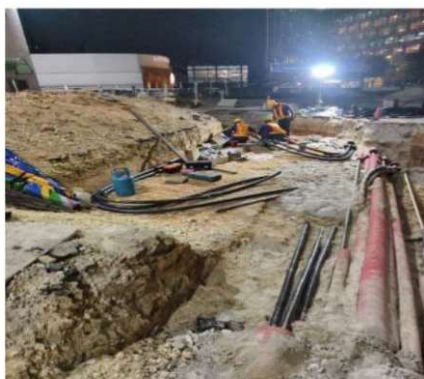
Figure 2: Laying Cable in Pipe
