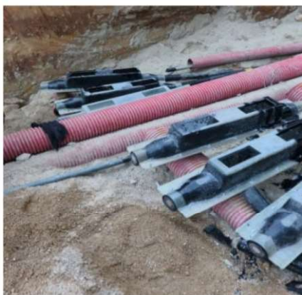
Figure 3: Joint Cable using Underground Cable Joint Kit
