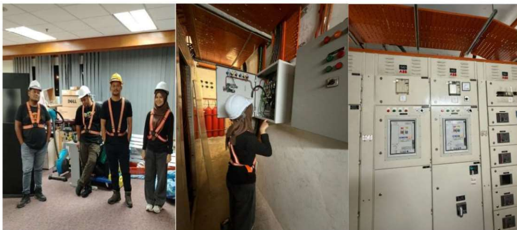
Figure 3: Site Work at LV Room at AMC Building, KLIA
