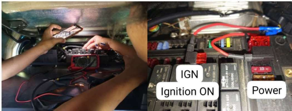
Figure 2: GPS Installation Activities at UPM
