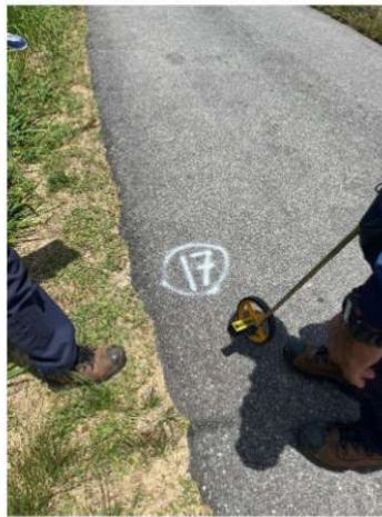
Figure 2: Distance Measurement for Installation of New Feeder Pillar
