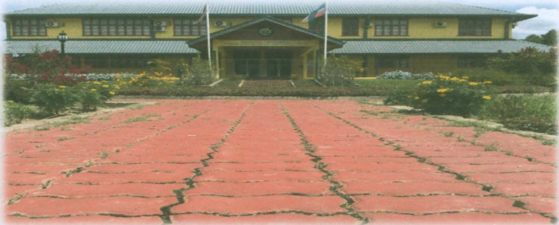
Figure 1: Main office of Tenom Agriculture Research Station.
