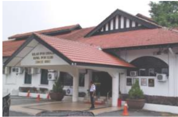
Figure 1: Front elevation of Royal Ipoh Club building
