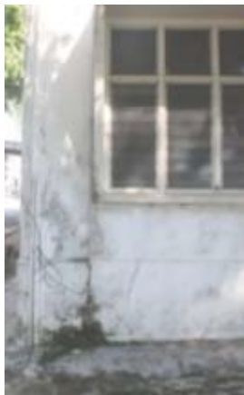
Figure 4a. Mould growth
