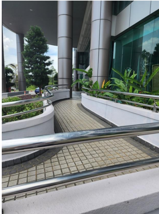
Photo 5.6: Ramp for wheelchair
