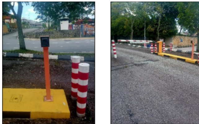
Figure 1. 21: Security gate barrier
