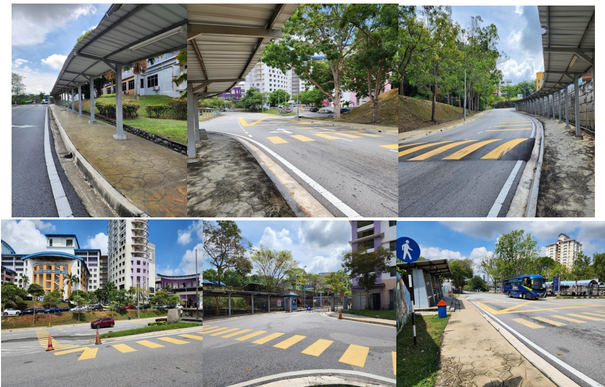
Photo 5.4: Covered walkways and pedestrian crossings
