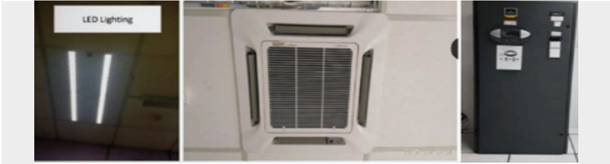
Energy Efficient Appliances being installed in most of buildings in UiTM
