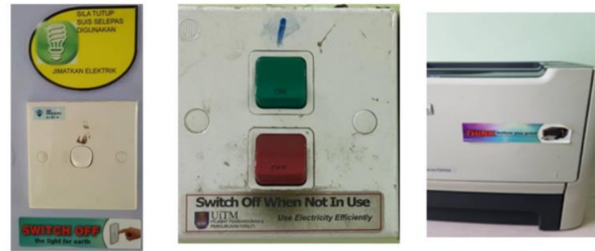
Figure 34 Awareness program on energy usage for switching, lighting and electrical appliances
