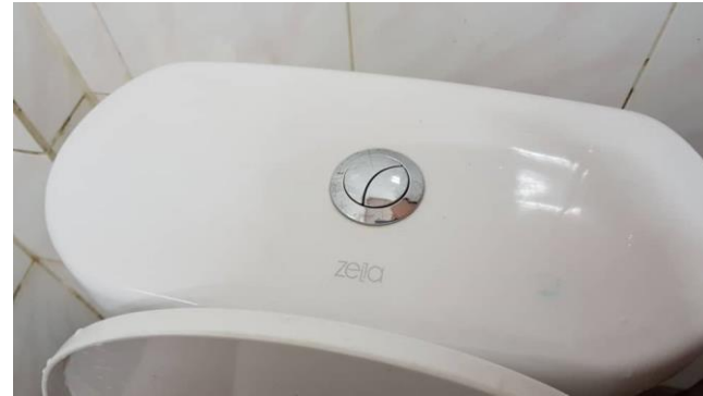
Figure 27 Install low and dual flush model
