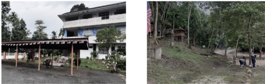
Figure 3: Before solar lighting installation in previous project
