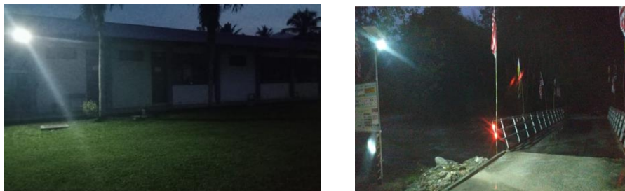
Figure 4: After solar lighting installation in previous project
