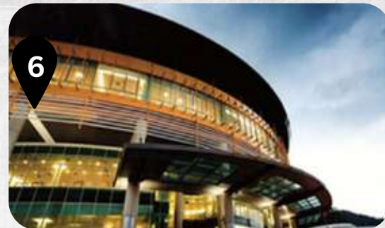
PTAR Kampus Selayang
