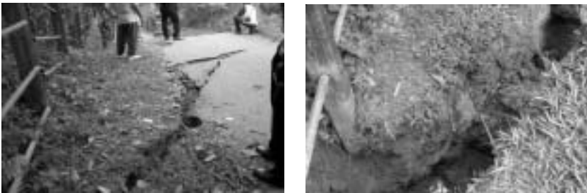
Figure 2: The development of tension crack at the crest of slope surface in which the present of rainwater will expedite the potential slope failure. Picture was taken at Wangsa Maju, Kuala Lumpur
