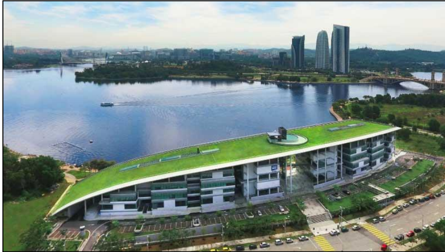
Fig. 1. Extensive Green Roof at Heriot-Watt University
