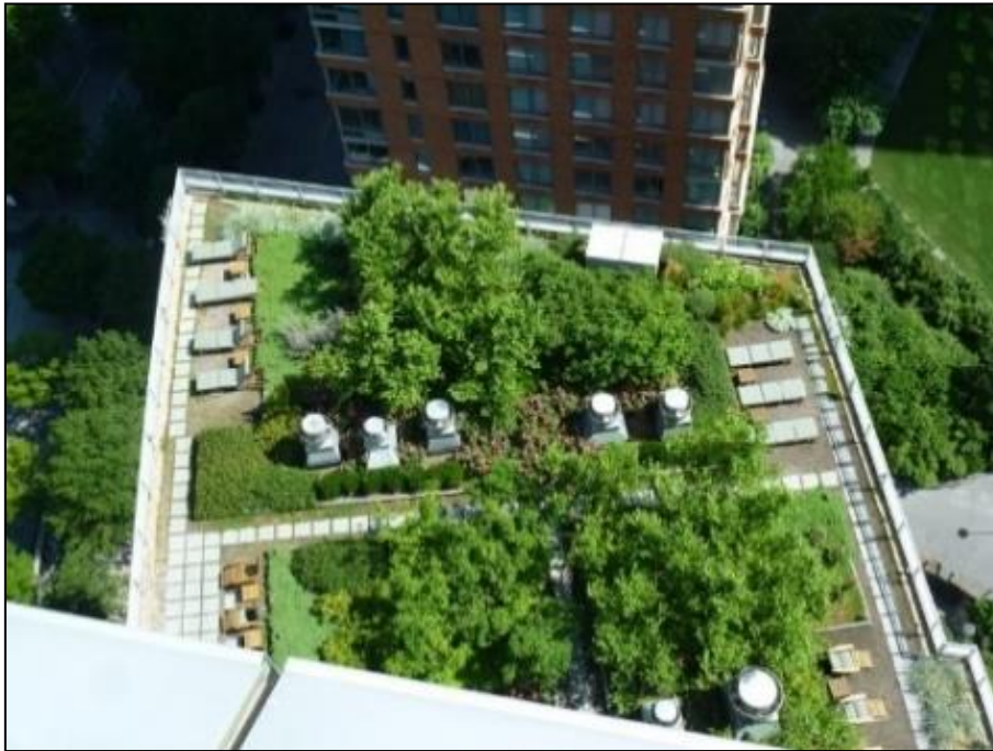
Fig. 2. Intensive Green Roof at Manhattan High Rise Building
