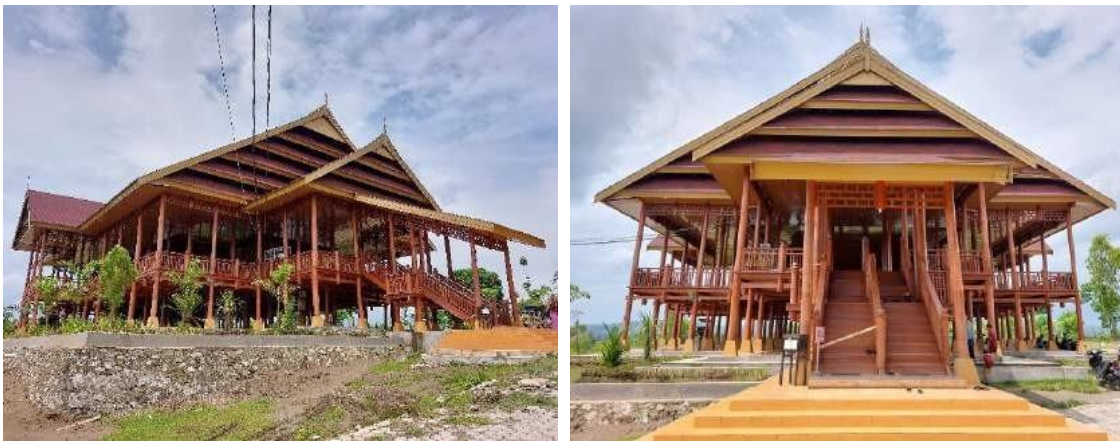
Figure 6 View of Boyang Kaiyang Art Studio, Survey (2023).
