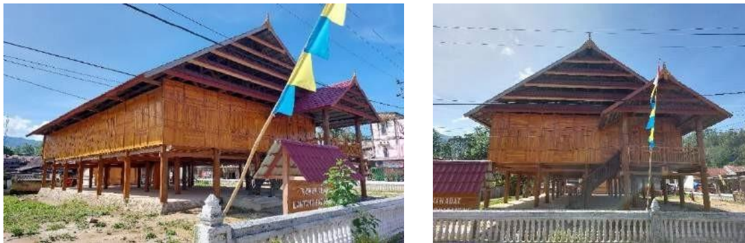
Figure 4 View of the Lantang Kada Nene Mambi Traditional House, Survey (2023).
