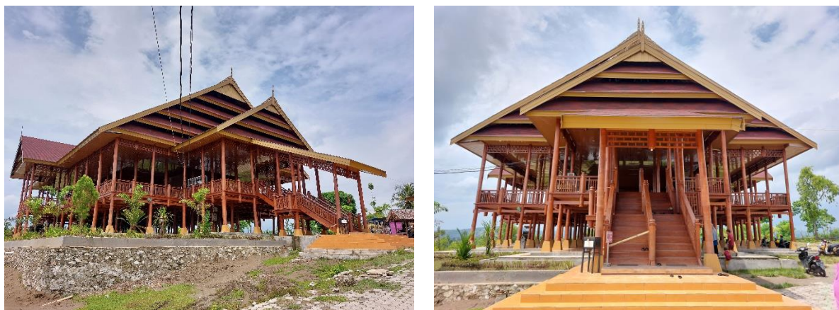
Figure 2 View of Boyang Kaiyang Art Studio, Survey (2023)
